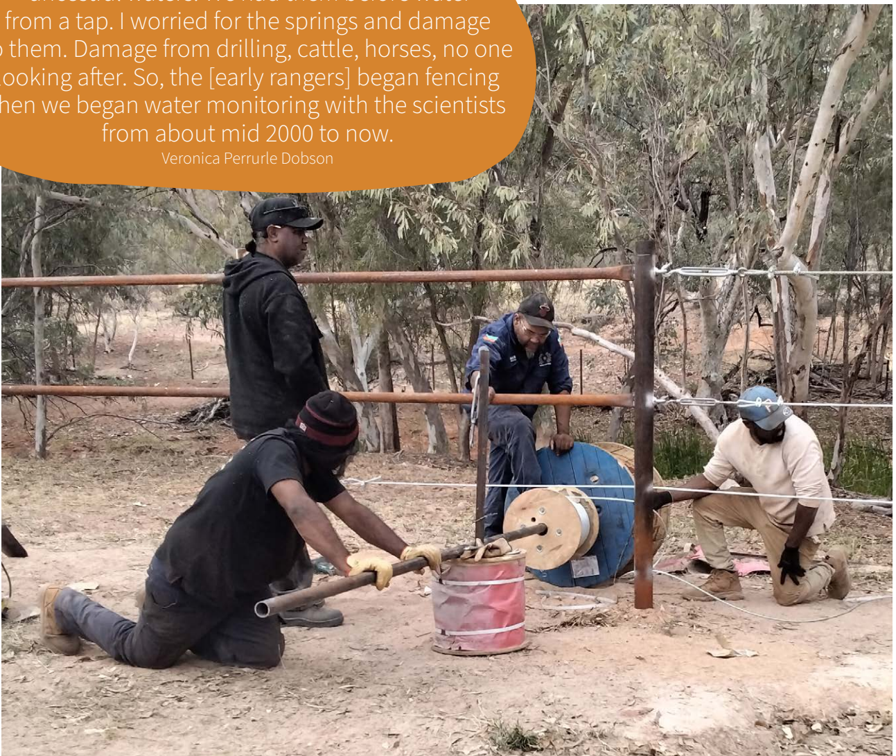
Rangers building a fence at Oolera Spring.
