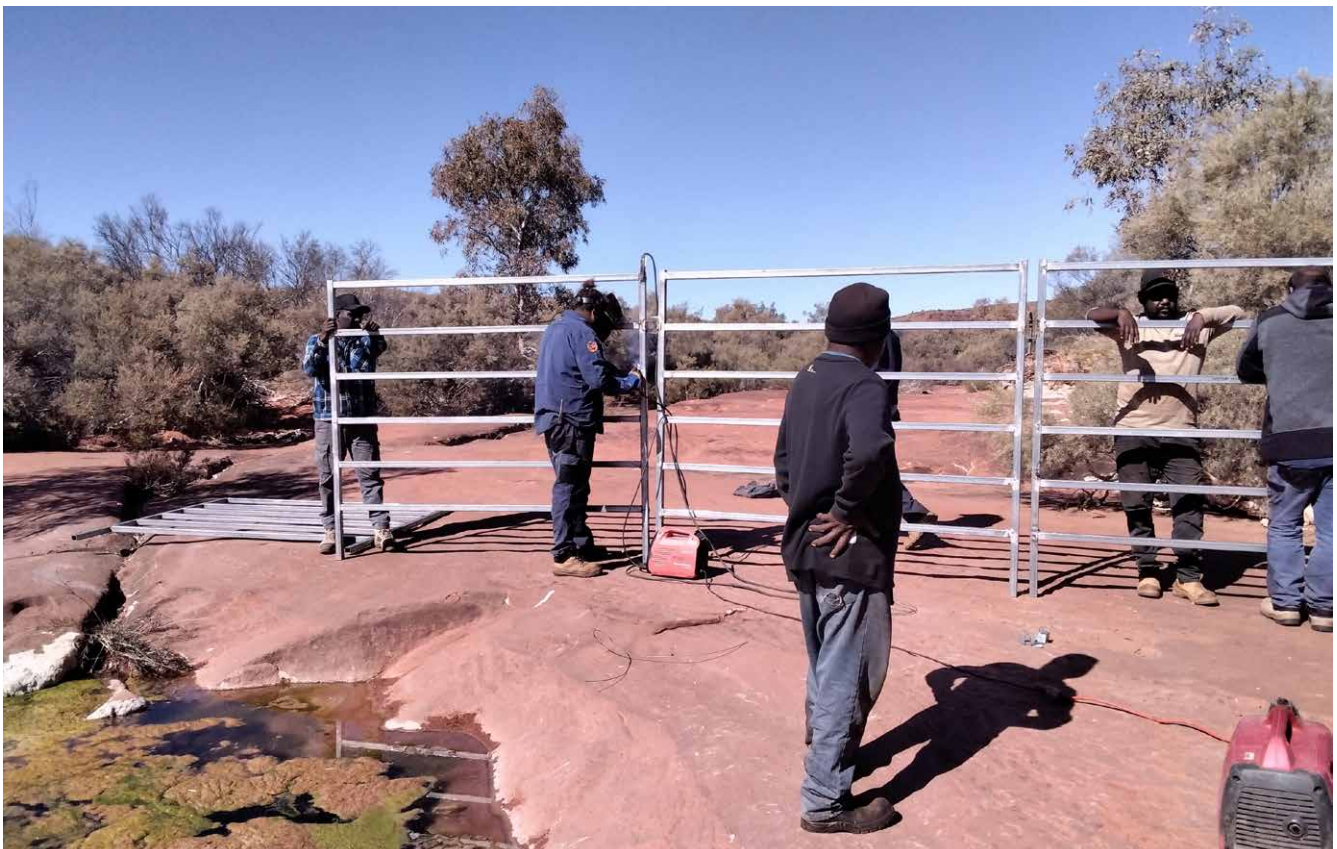
LEFT Patrick Abbott set up steel panels to protect a spring.
