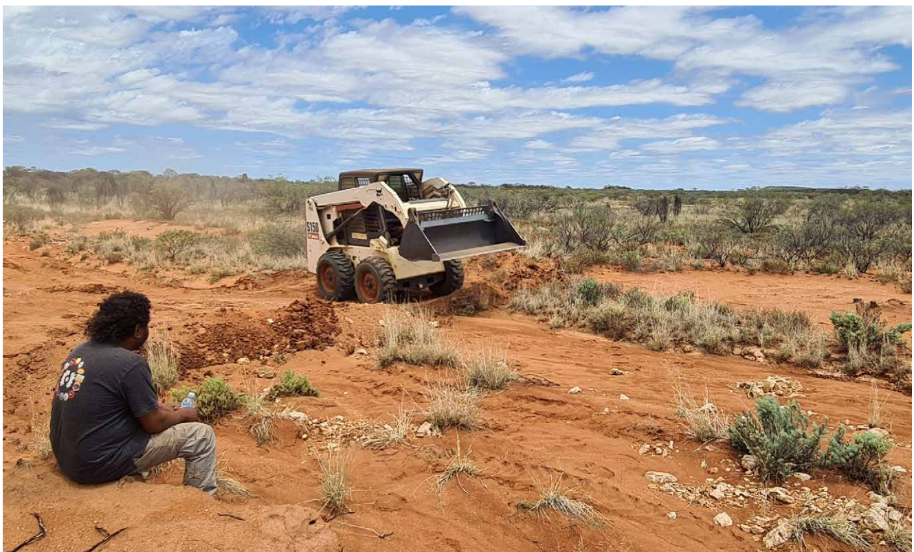
Anmatyerr Ranger Bevan Pepperill supervises while Maurice Campbell uses the bobcat to create erosion control banks on Ahakeye Aboriginal Land Trust.
