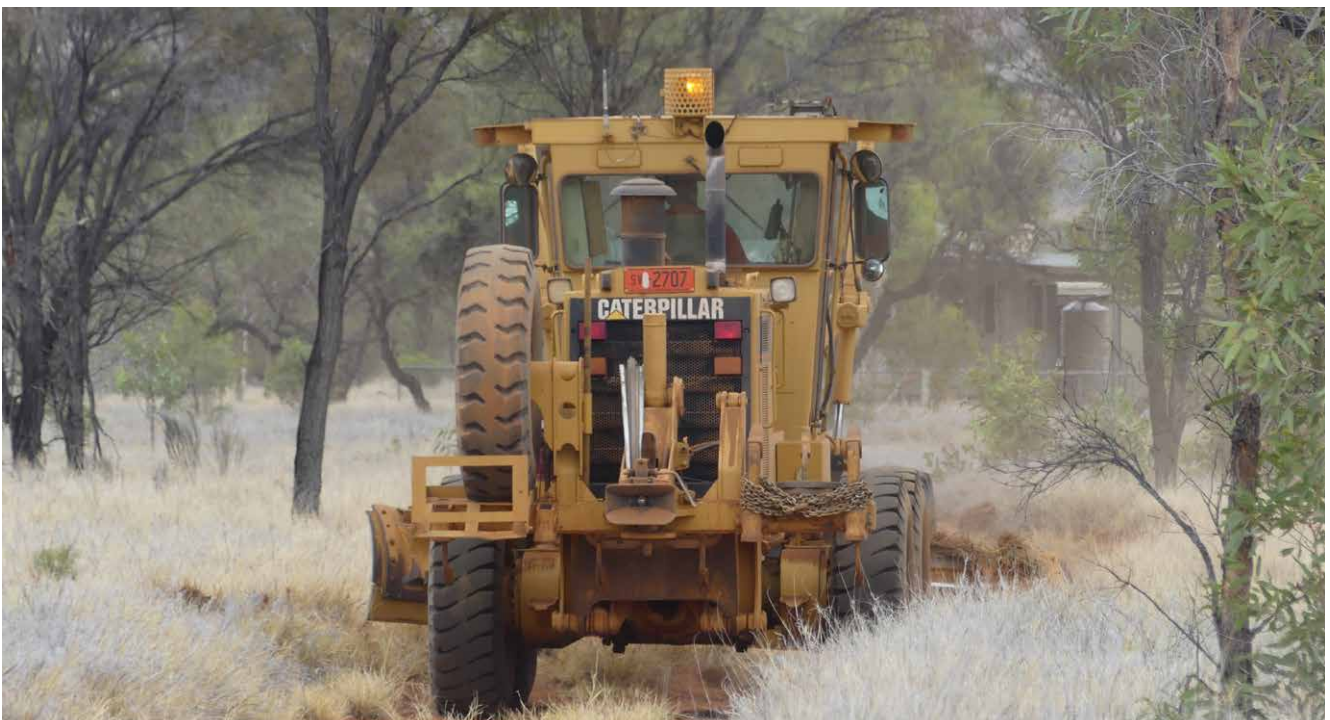
Grading the road to Eagle Valley outstation.
