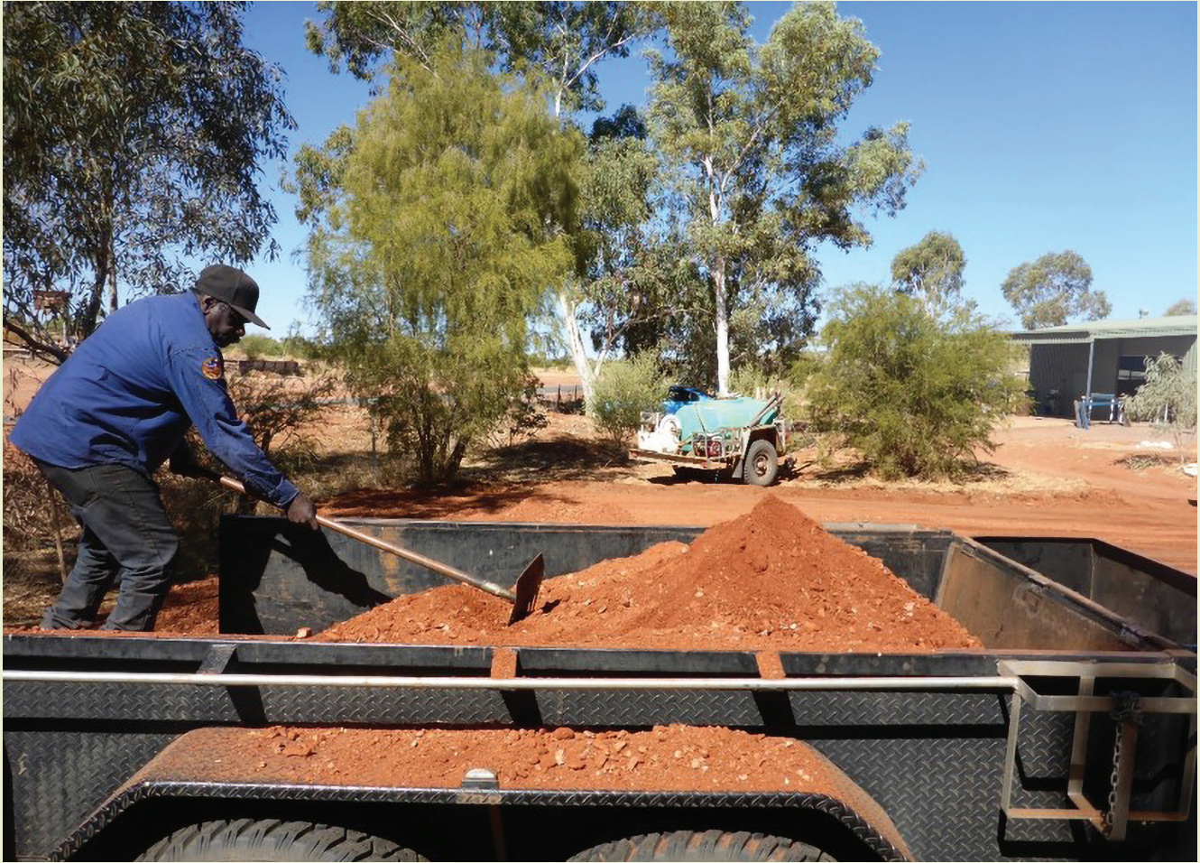
Christopher Ungwanaka working on new car park.
