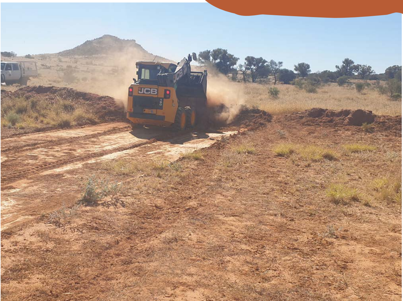
Use of Bobcat to repair erosion control banks on Santa Teresa Land Trust.
