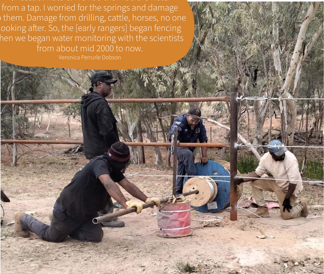
Rangers building a fence at Oolera Spring.
