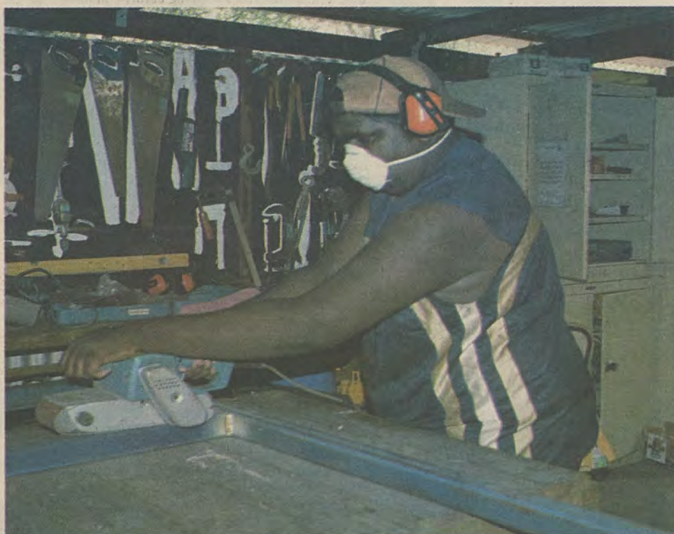
Above: Clinton Katarinja preparing an end-assembly for campground fencing.
