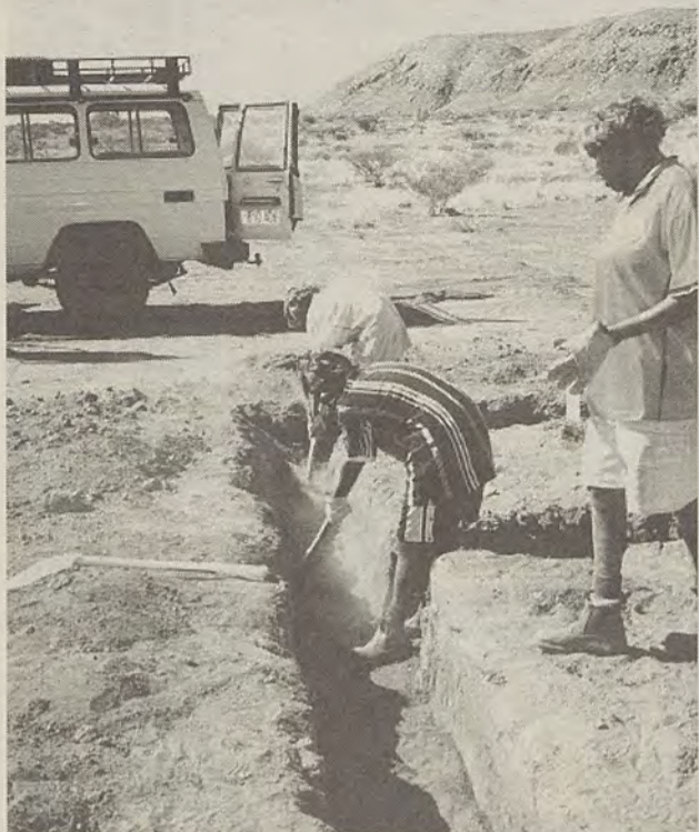
Digging footings - Evalissa Gibson and Judith Rowe
