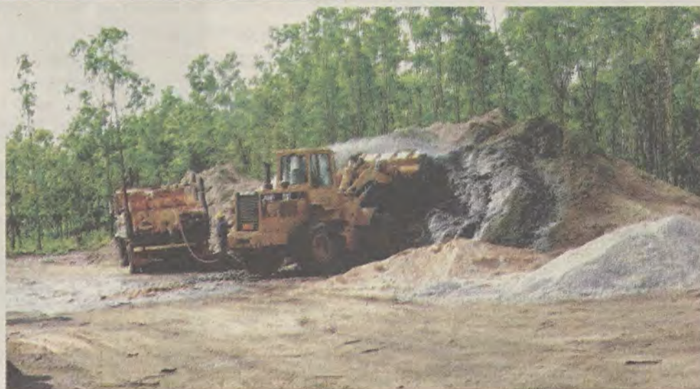
Work is well underway at the Darla site
